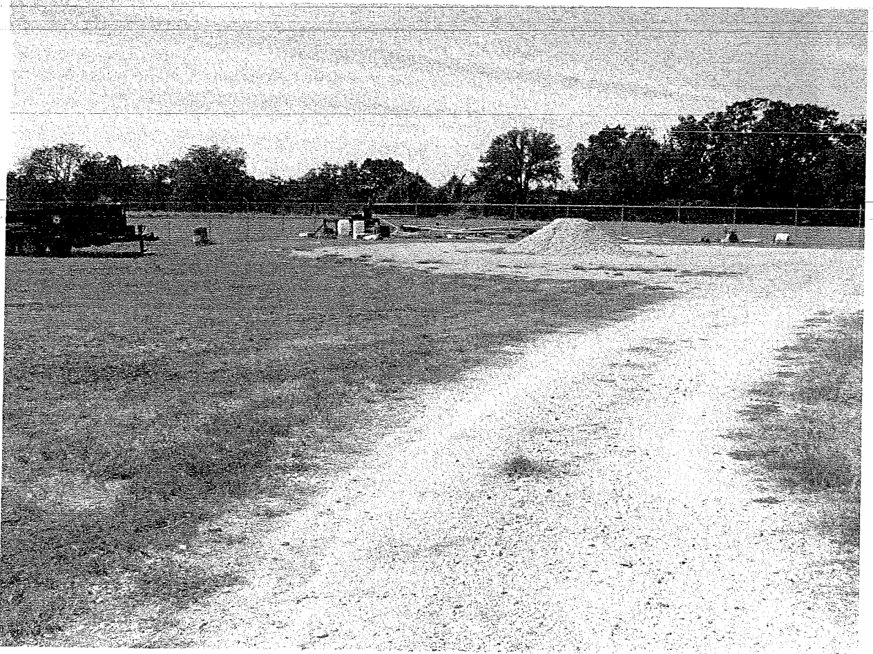
Picture 4 - Looking Southwest at Future WWTP and Effluent Filter Location (11-12-15).
